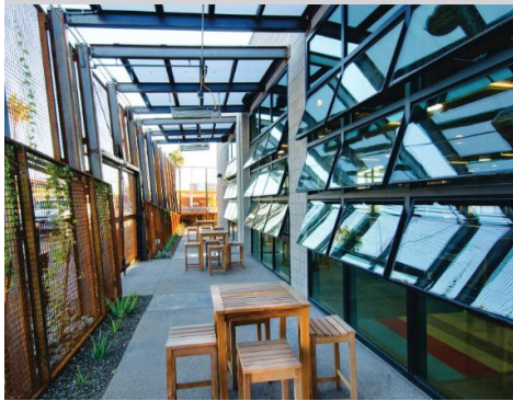
Figure 22: 87 operable automated windows
