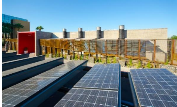
Figure 23: Photovoltaic panels are tilted 10 degrees.
