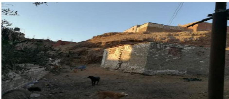
Figure 13: Houses on top of the site of Sandala, highlighting the lack of services (Accessed in 7/12/2023)
