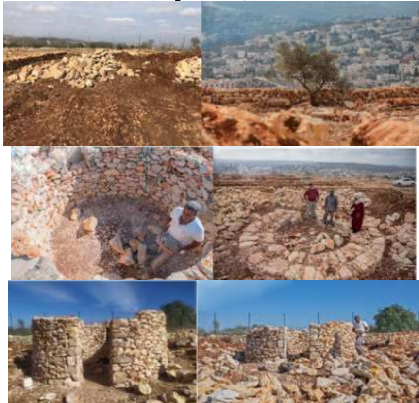
Figure 3. The construction process generally follows these steps. Source Muqaddi, Ala. (27-9-2020 )
