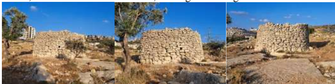
Figure 4. Al Rehan Area/ Ramallah City Al-Muntar in this region varied in shape. The simplest one is circular and has one floor and was built of random stones. Source author 2023
