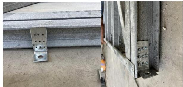
Figure (4): Hold Down Fixation with back-to-back Stud on Laboratory.
