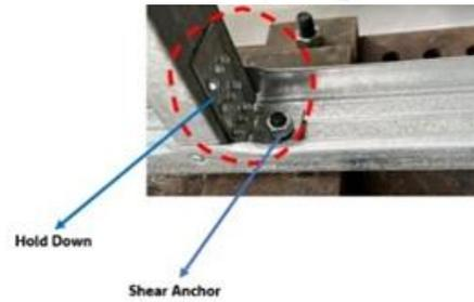
Figure (14): Shear wall frames details before sheath.
