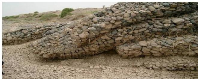
**Figure 9: Mitigation of flash flood using spur dike.**
