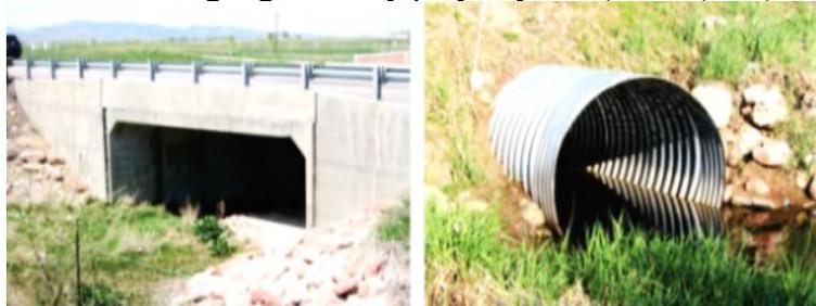
**Figure 11: Concrete box culvert and corrugated metal pipe.**
