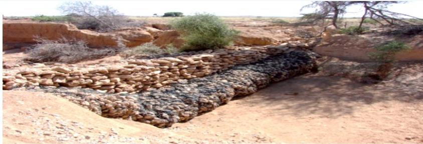
**Figure 12: Harvesting of Rainwater using gully plug**
