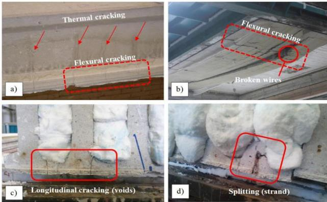
Figure 11: the cracking type
