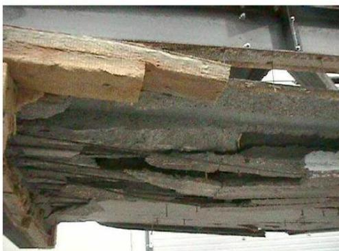
Figure 9: HCS Slab failure after fire [5]
