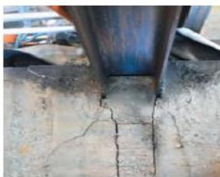
a Cracking around internal edge column
