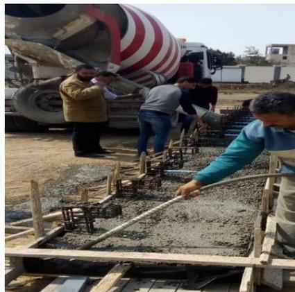
Fig. 4 Concrete casting-in-situ.
