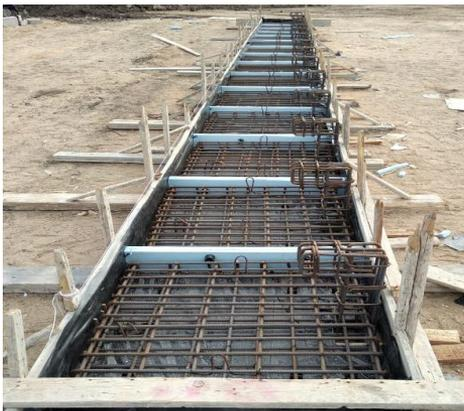
Fig. 3 Preparation form work and reinforcement.
