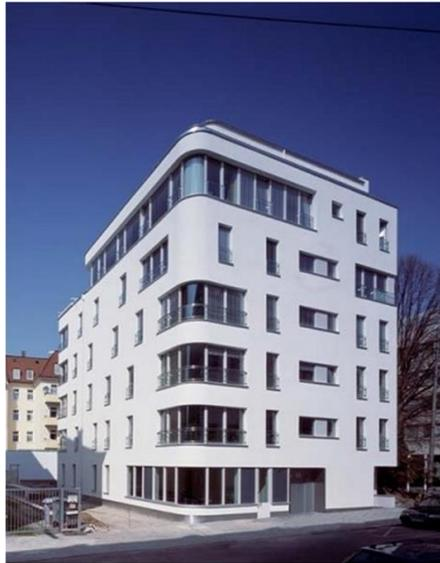
Fig.7 The Seitzstraße apartments with Vacuum Insulated Panels.
