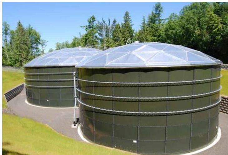
Fig. 2 Ground-level municipal potable water storage tanks [7].
