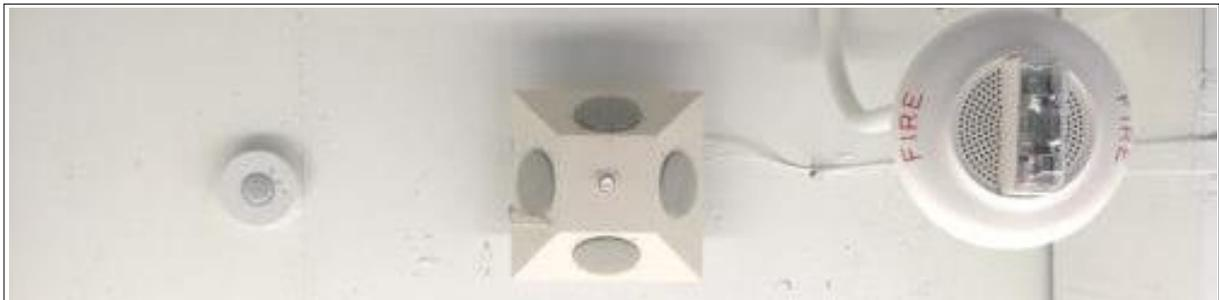
*Figure 20, Shows the ceiling where the sound masking system is installed in ASID headquarters office. (Source: Architectural Health/Yan Architects LLC, 2019)*
