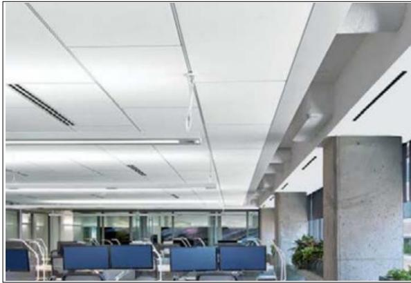
Figure 21, The suspended ceiling system consists of acoustic tiles absorbing sound in ASID office (Source: Armstrong®, 2018)
