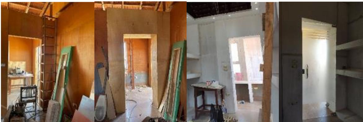
Photos n. (19) show the wall BB` before and after installing the wooden cladding, the initial paint stage, and after fixing the door.
