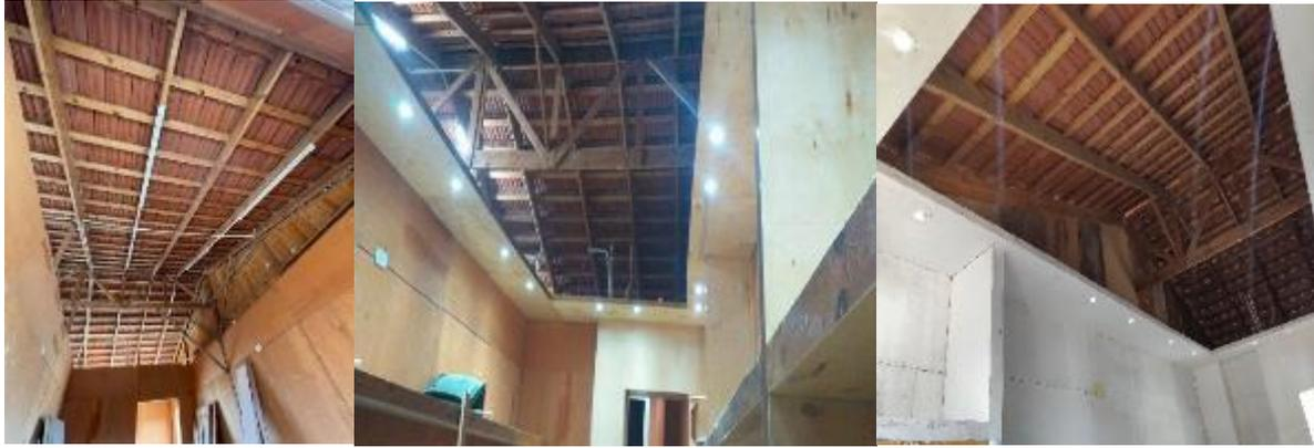
Photos n. (20) show the development of the ceiling before and after, the last one for the ceiling with lighting and initial paint.
