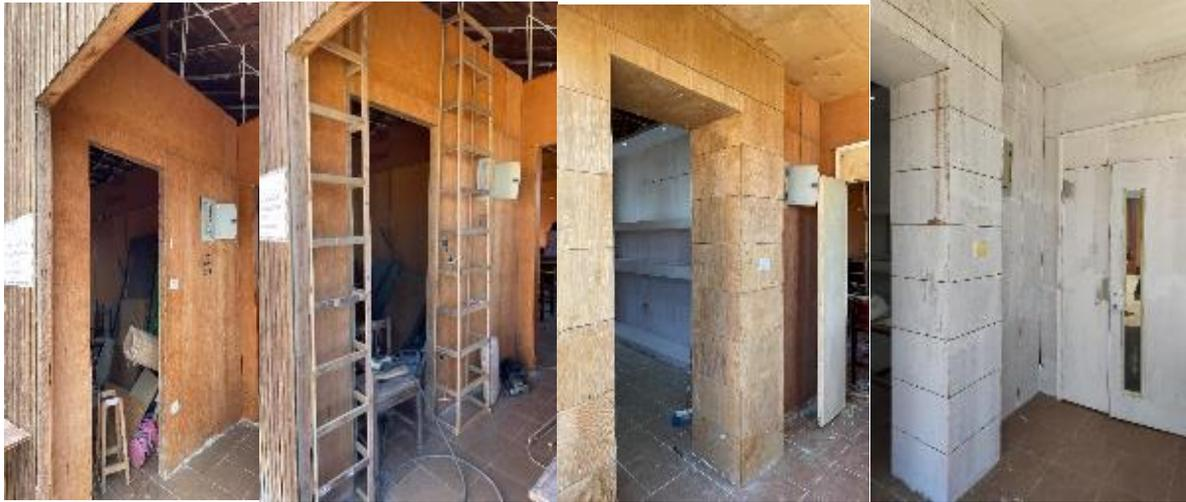
Photos n. (23) show the wall EE' before, though, and after fitting the wooden cladding. The last photo was in the initial paint stage.
