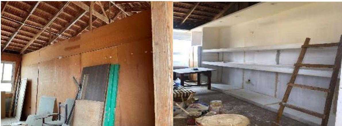
Photos n. (15) show the wall AA` before and after fixing the shelves that will carry the displayed pieces of furniture, the storage unit, and the desk. The second photo was in the fixing shelves stage.
