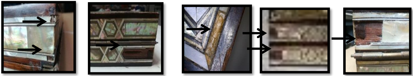
Figure 7 Loss of some inlaid units
