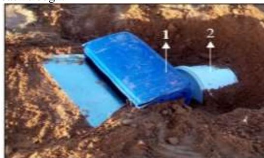
Fig. (5) Trough used for collecting rainwater runoff.
