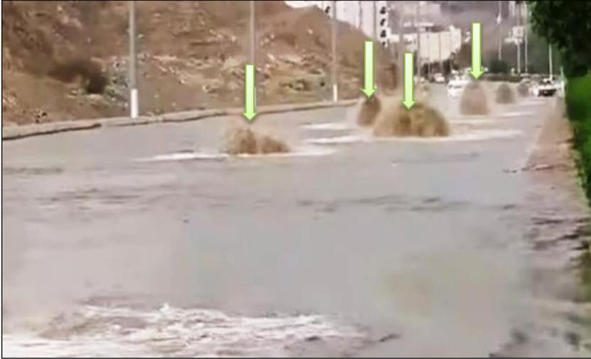
**Figure (31): Photograph shows the poor absorption of the flow drainage network and the exit of water from the main hole.**
