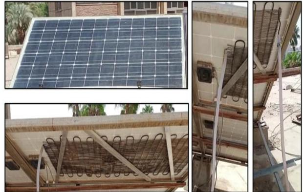
**Fig. 10** Iron-serpentine with water technique for cooling PV Panels (Panel C).
