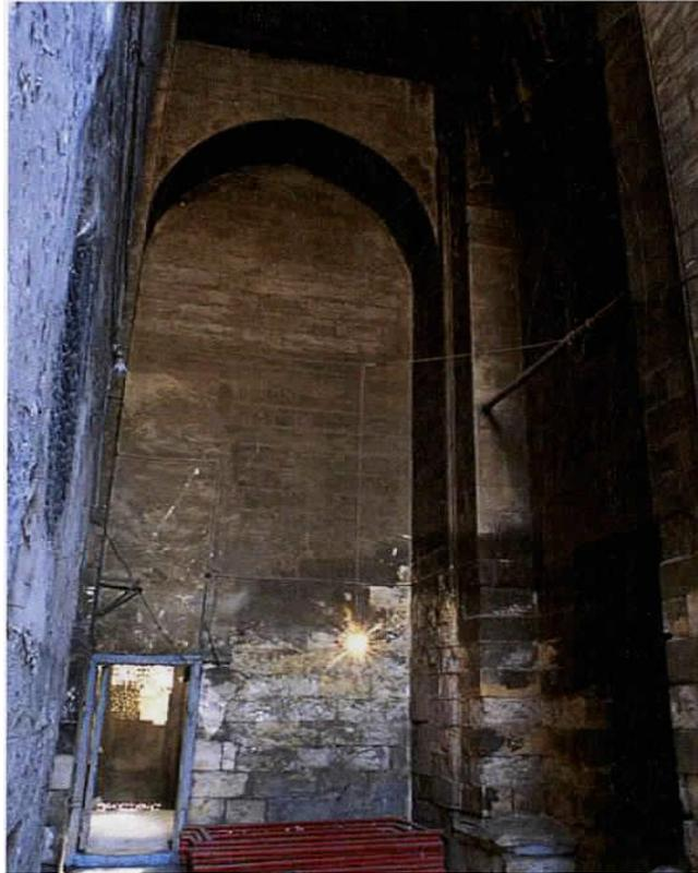
Plate 13. Madrasa of Umm al-Sultan Sha'ban, construction joint between Sabil and inner portal
