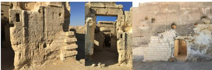
Figure 6: Some of the restoration work to complete the walls of the Temple of the Oracle, which were destroyed due to the erosion and weakness of the original limestone walls. ©
