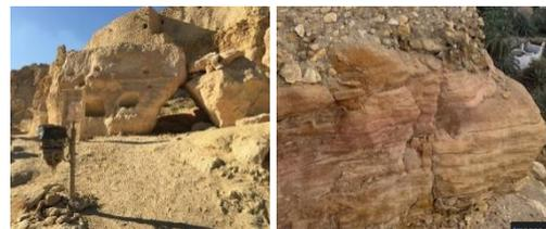
Figure 7: Manifestations of erosion and cracking of the Aghurmi rock, which threatens the safety of the temple and other ancient buildings. ©
