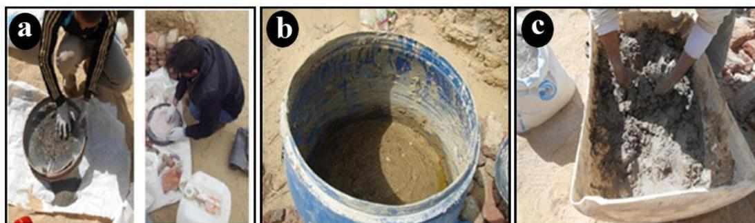
**Fig. 10. Stages of preparing the mud mixture for manufacturing mud bricks, and preparing the mortar mixtures used in different restoration works (a) Sieving the ingredients and purify them from impurities, (b) Fermentation process, (c) Kneading process.**
