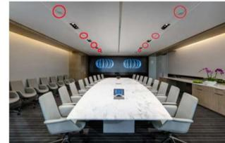
Fig.34 The Occupancy sensors and the Control Tablets [43].
