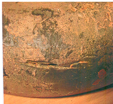
Fig. 18. Slit formation in a reheater tube due to creep.
