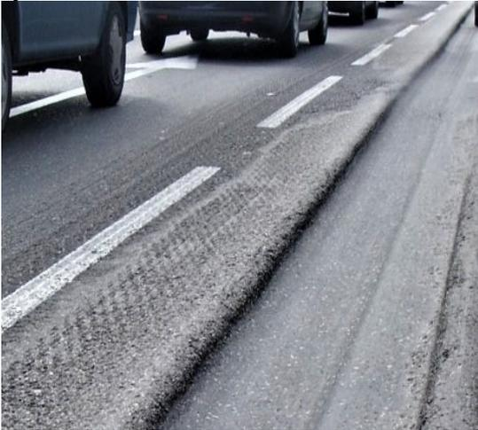
Fig.(1)Permanent deformation (Rutting)
