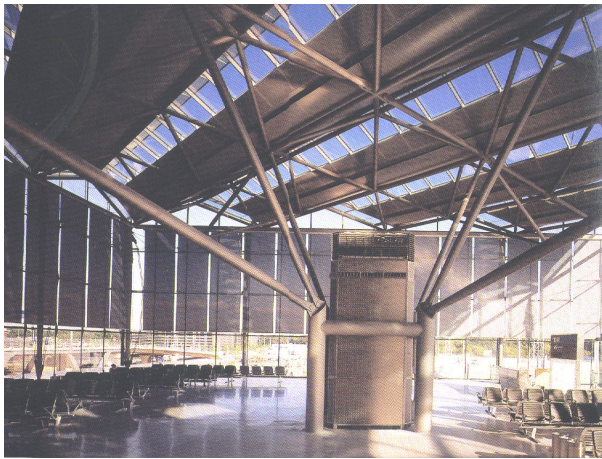
Structure tree columns with large clear spans accommodating Services equipments Terminal 2 Cologne - Bonn Airport Germany [R3]
