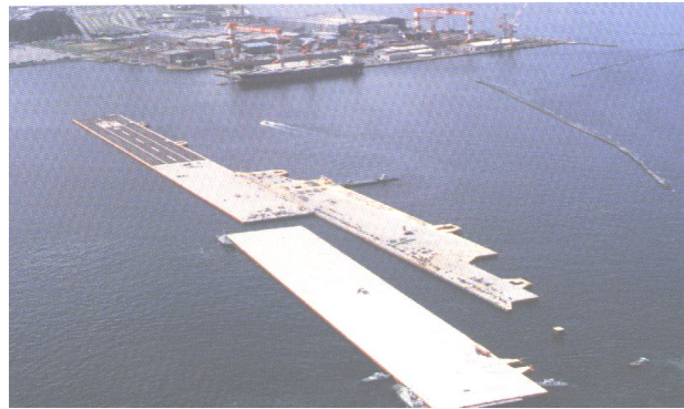
The working prototype of Mega float is assembled In Tokyo bay - at 2000 [R4]
