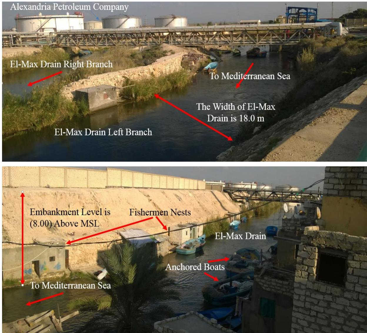
Fig. 3. The DR's embankments, fishermen's nests, tethered boats, and oil company bridges on January 6, 2016.
