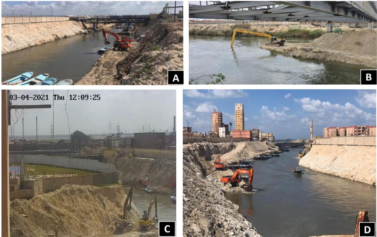
**Fig. 14.** A) and B) Obstacles in implementation, objections to the bases and foundations of the bridges of the oil companies; C) and D) The contractor encountered difficulties in implementing the 180-meter dredge near a sports club wall on the right bank of the drain path.
