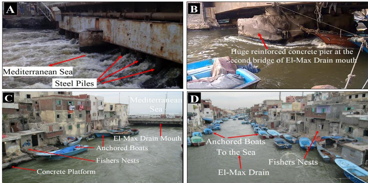
**Fig. 4.** Restrictions along the El-Max Drain path: (A) water level rising caused by steel piles filled with plain concrete at the mouth; (B) channel throttle caused by a large reinforced concrete pier at the second bridge at the mouth; (C) and (D) channel throttle caused by anchored boats, concrete platforms, and fisherman's nests on January 6, 2016 [1].
