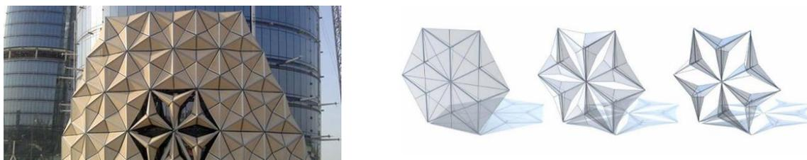
**Fig. 2: Al Bahar Tower - Smart Facade System.**
