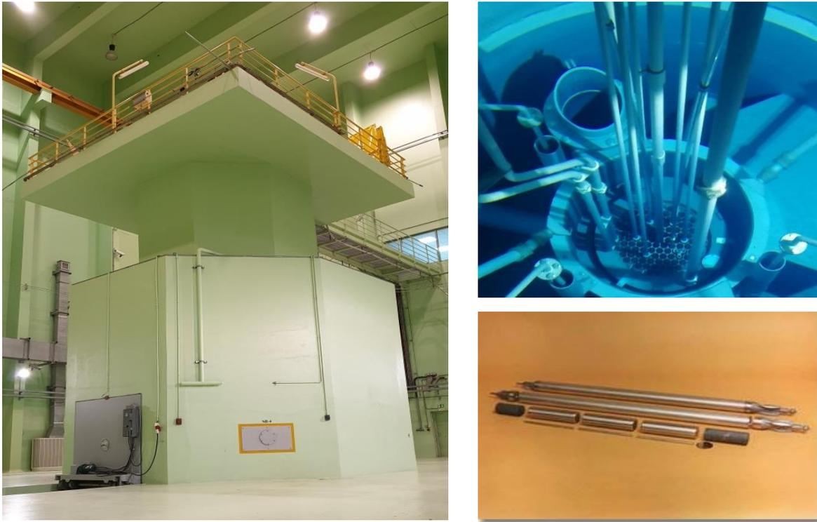
**Fig. (1): Experimental Hall and reactor bloc (left) / TRIGA fuel elements and Reactor core (right)**
