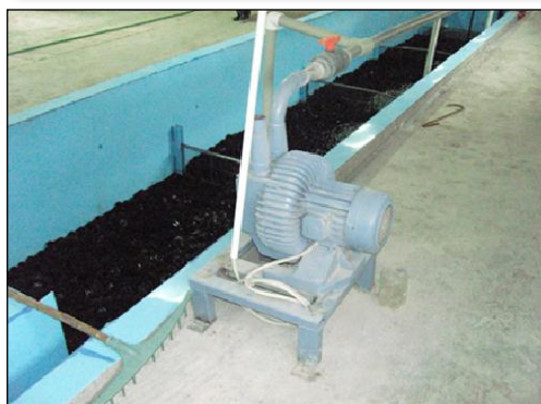
Fig.4. Aeration system of the biological filter (Lazaet al. , 2021)
