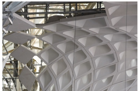
Fig. 4 GFRC architectural cladding
