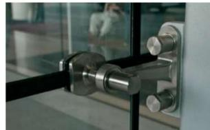
**Fig.7** Point fixed clamped system (Patterson, 2011)
