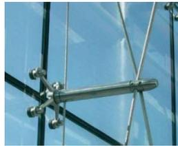
**Fig.6** Point fixed bolted system (Patterson, 2011)
