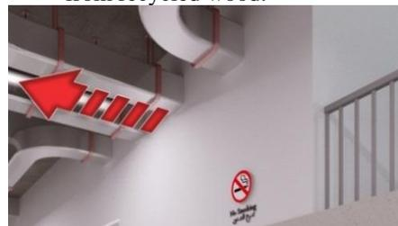
Figure 39: Air ducts exiting the service skylight and distributing them to the right and left of the classrooms and administrative spaces.
