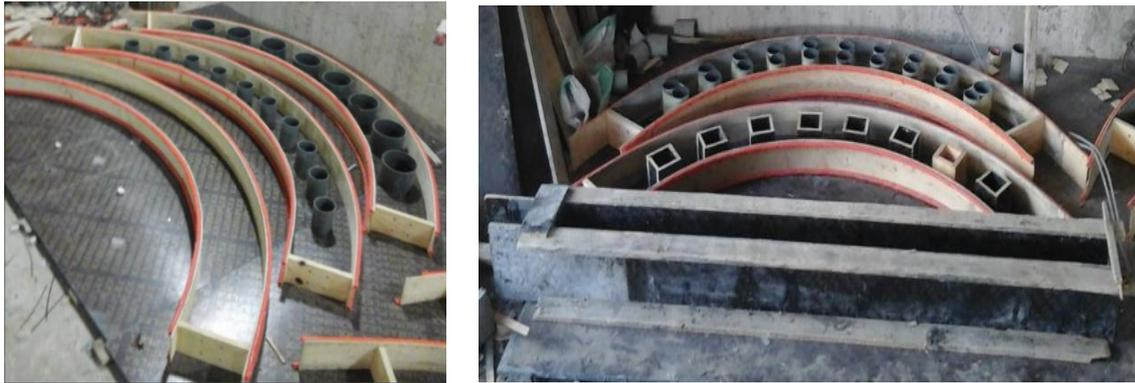
**Fig. 3 Formwork used for casting BSS, BCS-C-R60, BCP-D10-R60, BCP-D20-R60, BCP-D15-R60, BCP-B15-R60 and BCP-O10/20-R60.**
