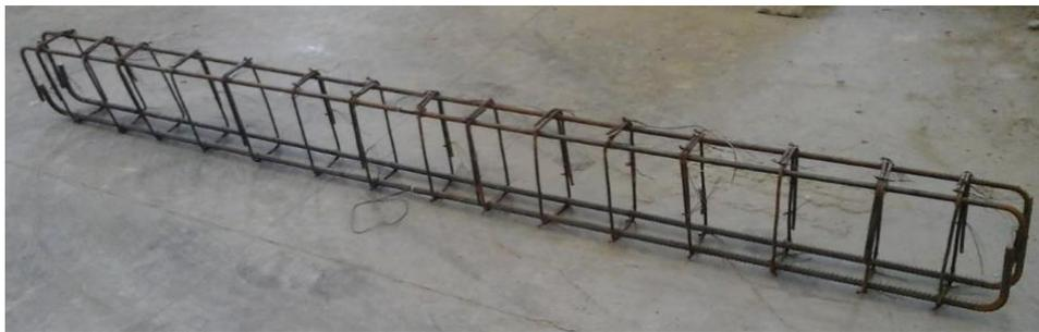
**Fig. 4(a) Reinforcing steel cage of BSC.**
