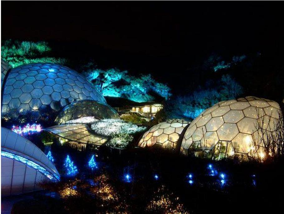
foil) suspended on steel structures to cover 2.2 hectares, The construction of the design was based on the most stable forms on the ground while providing maximum strength with minimum materials. The interior of the domes provides different growing conditions for plants, and the multiple domes of each have a different environment from the other as can also be seen on the screens installed inside, For example, a tropical dome
