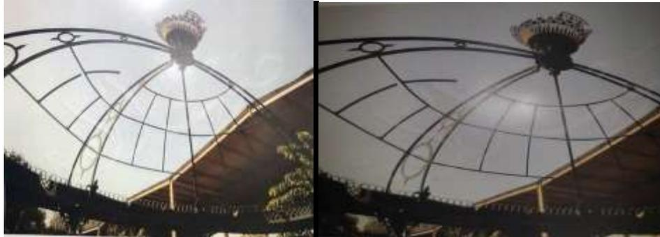
*Figure 26: The remains of the dome's circumference with its metal beams of the music kiosk in Cairo's Azbakeyah garden (By the researcher)*
