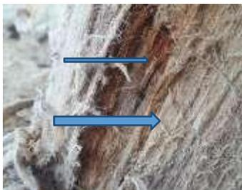
**Figure (1-1)** shows the bottom window frames of one of the windows of the coastal corridor of Qaitbay Castle. The figure shows the fragmentation and separation of the wood surface and the accumulation of salts because its proximity to the sea.
