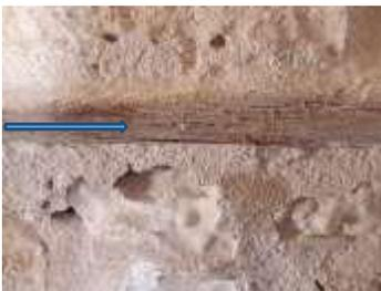
**Figure (1-2)** shows one of the wooden beams inside the sandstone wall on the floor. The wood surface is damaged and the fiber is broken by the salts and the resulting pressure.
