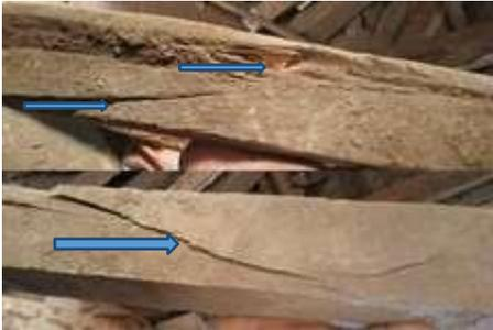
**Figure (5-2)** The wooden beams from the ceiling have mud brick residues and suffer from loss in some parts, cracks, breakings, horizontal shear, and compression and cross grain tension.
