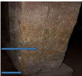
**Figure (1-3)** shows one of the wooden pillars inside the tombs of Kom Al-Shaqafah, which suffer from biological damage, crushing, splitting and cracks resulting from the pressure on it.
