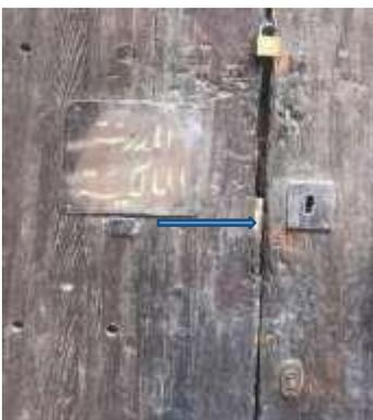
**Figure (3-2)** from a door in El Soltan Hassan school shows that the wood suffer from height humidity, biologic deterioration and defiberation.
