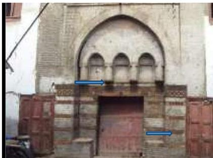
**Figure (5-1)** The main facade of the Jaddawi Agency shows the overlap of wood "wooden beams" with the building materials such as brick masonry, black cement, and mortar layer of lime, in addition to mud bricks.
