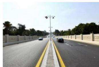
Figure (12): El-Merghany Bridge shows El-Orouba intersection with a length of 550 meters and a width of 21 meters, and includes 3 traffic lanes in each direction - Source: Egypt Projects Map website.
