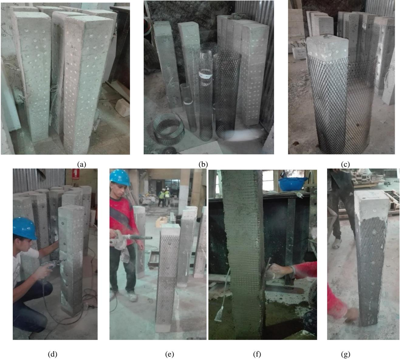
Figure 4: Strengthening procedure for jacketed specimens
