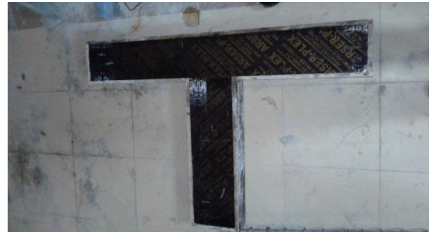
Figure 7. Form works that used for casting
