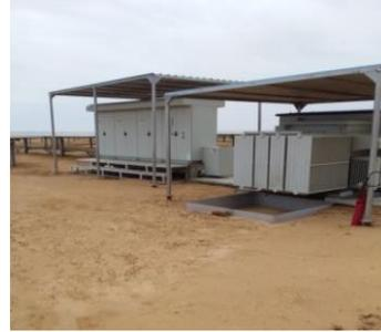
Photo.5. Inverters and transformer
