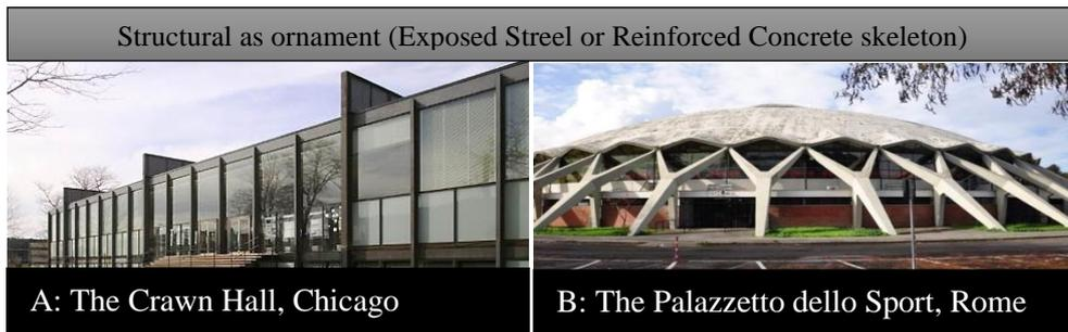
Fig. 4: A) The exposed steel skeleton, including the plate girders that rise above the roof was used as source of ornamentation in the Crown Hall, Chicago, USA, 1952-56, by Mies Van Der Rohe. B) The exposed inclined exterior reinforced concrete struts were used as source of ornamentation in the Palazzetto dello Sport, Rome, 1957, by Annibale Vitellozzi, Source: A: [3]; B: [42] respectively.
