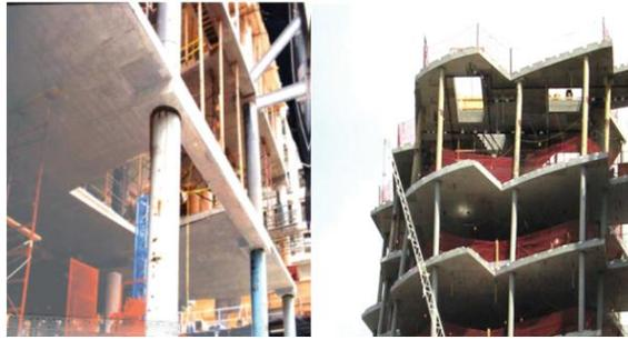
**Fig. 1.** Large Opening in Flat Slab Floor [1].
