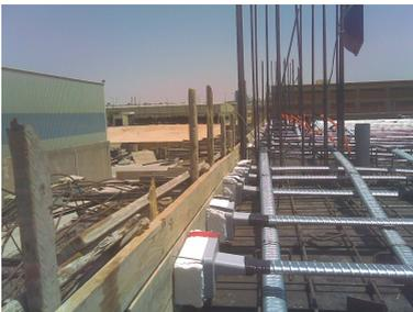
**Fig. (10): Tendons passing through interior column**
