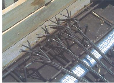
**Fig. (11): Tendons passing through exterior column**
