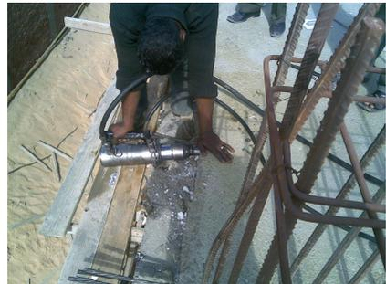
**Fig. (26):** Tensioning process
