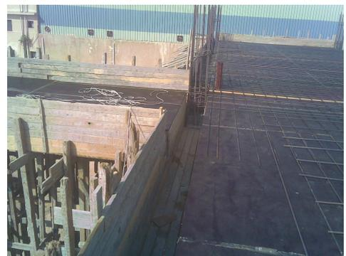
Fig. (6): Flat slab form
