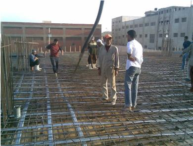
Fig. (22a): Concreting of slab
