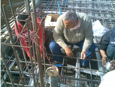
**Fig. (19a): Strain gauges at exterior column**
