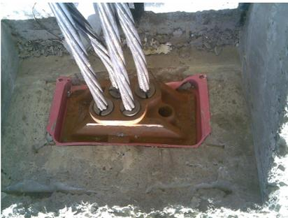
**Fig. (24):** Wedges in cast after tensioning of strand
