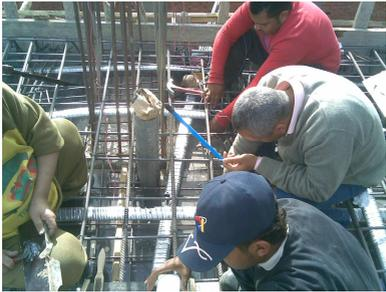
**Fig. (19): Box for tensioned tendons**
