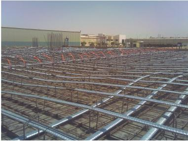
**Fig.(9): Tendons positioned in two directions**
