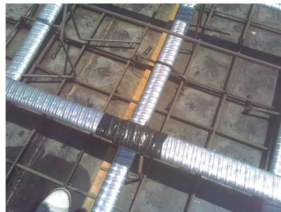
**Fig. (14): Plastic pipes for grouting**
