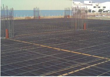
**Fig.(7): Bottom Non-Pre-stressed Reinforcement**
