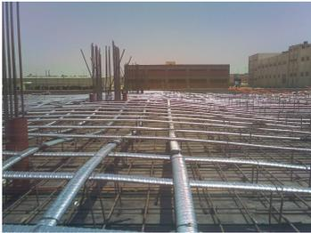
**Fig. (8): Tendons positioned in two directions**
