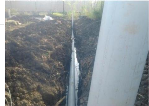
Figure 1: Burying of a pipe within the ditch
