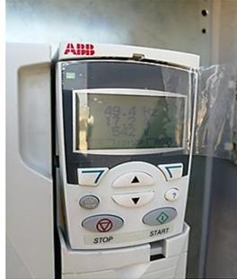
**Fig.(1): AC variable speed drive/ low voltage drive**
