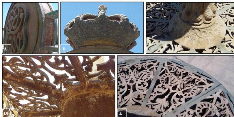
Fig. 2 A, B show the corrosion products on the surface of the bronze objects, C, D, E show the corrosion compounds and details of the iron table at King Farouk corner museum.
