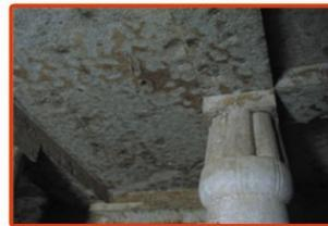
**Photo 5.** Effect of rain water at the ceiling and inside tombs at Bani Hassan.
