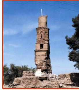
**Photo 2.** Effect of wind erosion at El Bahnasa site (Minaret Abu Samra).
