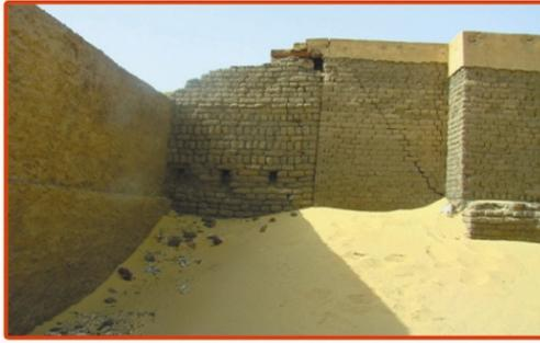
**Photo 1.** Failure and cracks in the walls catch tomb at Tuna El Gabal as a result of wind erosion on the foundation.
