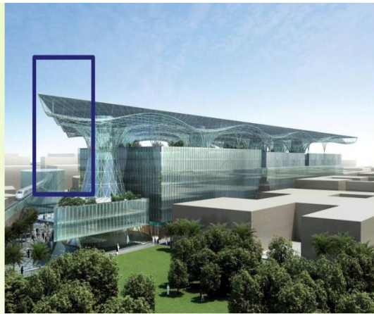
The use of metal structures and trusses, which have large prominence, enable shading
