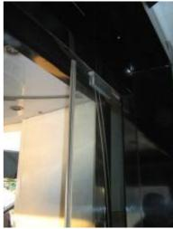
Picture 38 provided a break using rubber to reduce shock and friction resulting in cracking door leaf
