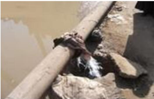
Fig 11: Pipes passing over waterways and leaking .occasionally- Kafr Hakim village, Geiza
