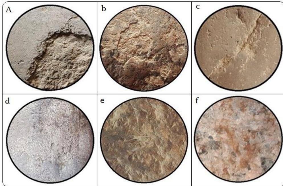
**Fig. 3. Deterioration aspects of the studied granitic columns. (a, b) scaling and granular disintegration of surficial layer at the lower parts of the granitic columns; (c) cracks and pits at the lower parts; (d) salty layer, pits and voids; (e) deposition of soot and dust on the surface; (f) spots of hematite.**
