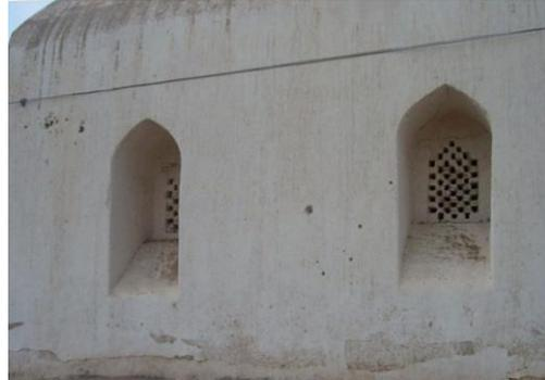
**Fig 6:** *Abutment walls which supported walls of Madrasa of Mustafa pasha in Zabīd.*
