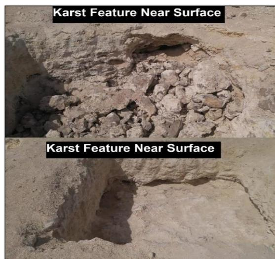
**Fig.3d.** Excavation near the surface in the Middle Sector shows a karst cavity at the boundary between Simsima and Khor members
