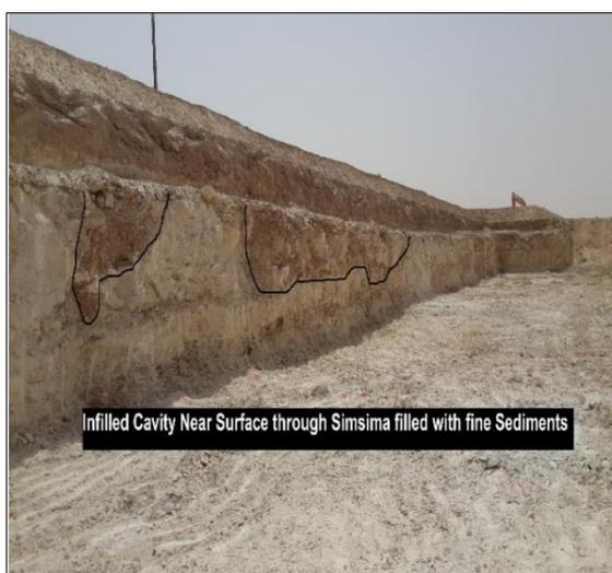
**Fig.3c.** Excavation cut near Al Khor, show filling of cavities in Simsima Layer by Quaternary deposits
